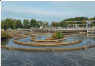
Waste Water Treatment
